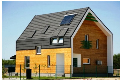
Fig. 1. The first serial energy efficient house in Ukraine
