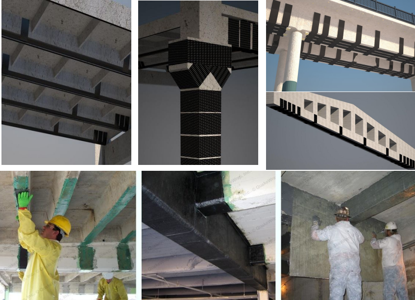
Fig. 11. Image representations the systems for strengthening of reinforced concrete structures by FRP-materials
